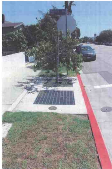
Grand Boulevard in Venice after installation of engineered tree wells.
